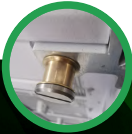
CABINETS SECURED BY POSITION PINS
